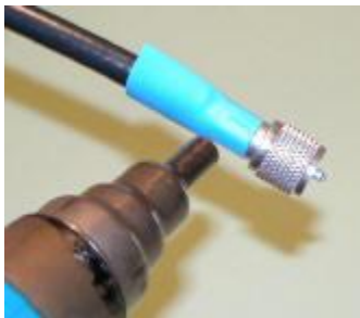
Step #11B With the right touch, the shrink tubing will run perfectly
